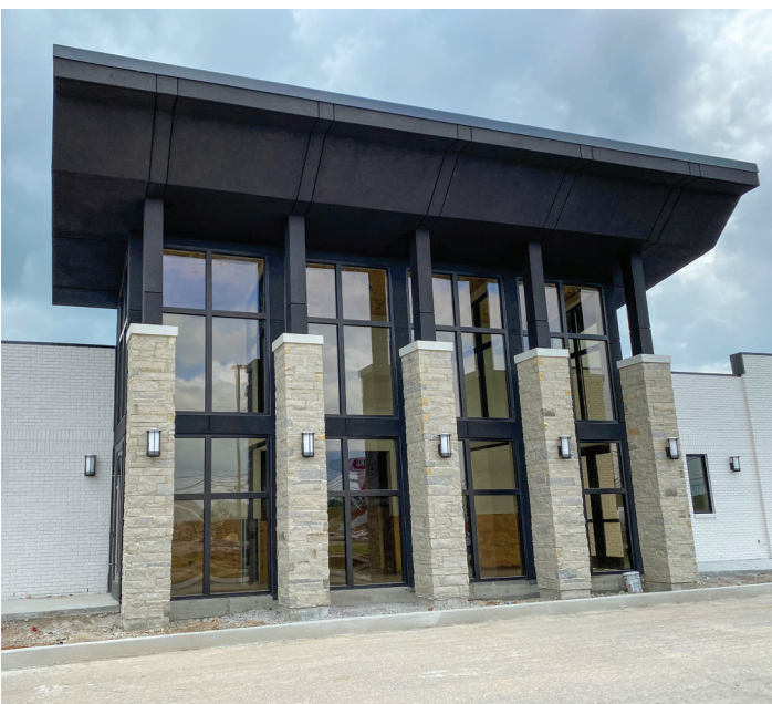
The exterior of the building features stacked stone columns, exterior insulation and finish systems (EIFS), and new paint.
