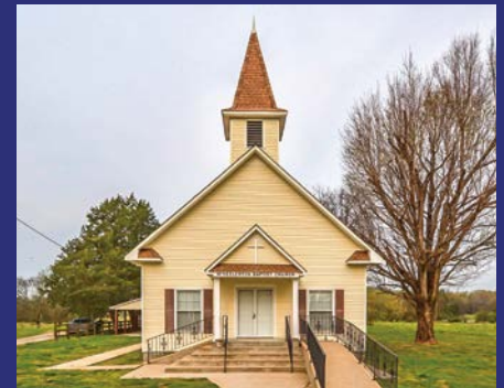
Construction began recently at Wheelerton Baptist Church.
