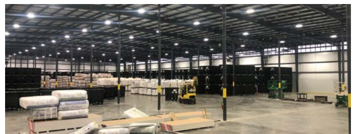
A new 100,000-square-foot warehouse was constructed for Allsource, enabling them to reopen in October 2022.
